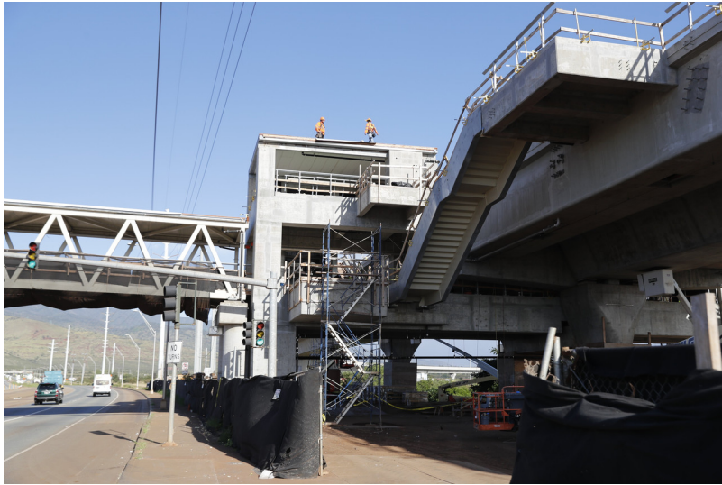
A rail station under construction in Kapolei in West Oahu.
